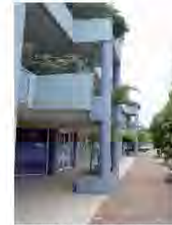
This colonnaded ground floor is not a good precedent for the village centre: it mitigates against the feeling of an open, inviting shopfront that is part of the public domain. It appears to discourage rather than encourage pedestrian movement next to the commercial entries.
