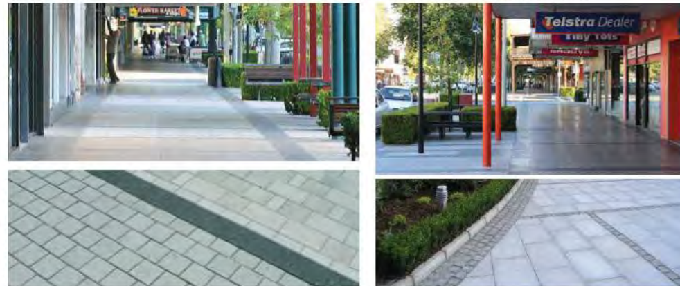
PEDESTRIAN PAVING - GRANITE BLOCKS IN GREY TONE AND DIFFERENT COLOUR BAND TO DIFFERENTIATE SPECIAL AREAS
