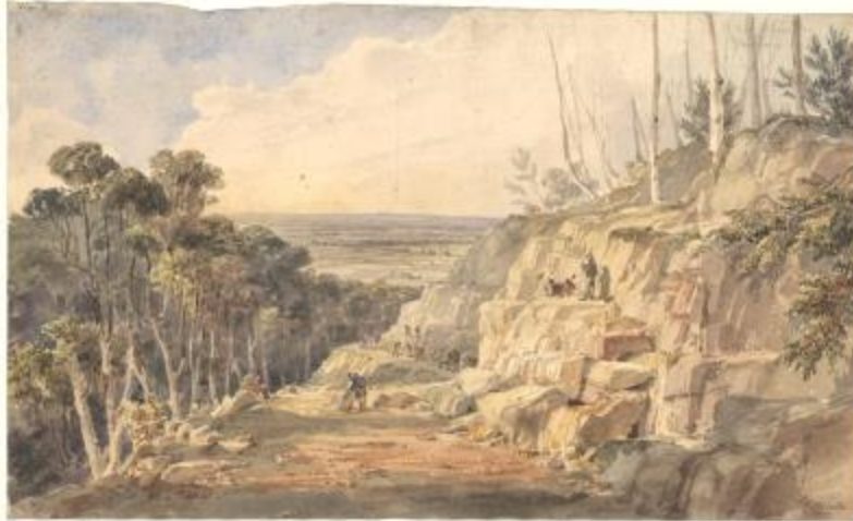
Convicts building road over the Blue Mountains, N.S.W. 1833. Charles Rodius. Courtesy National Library of Australia
